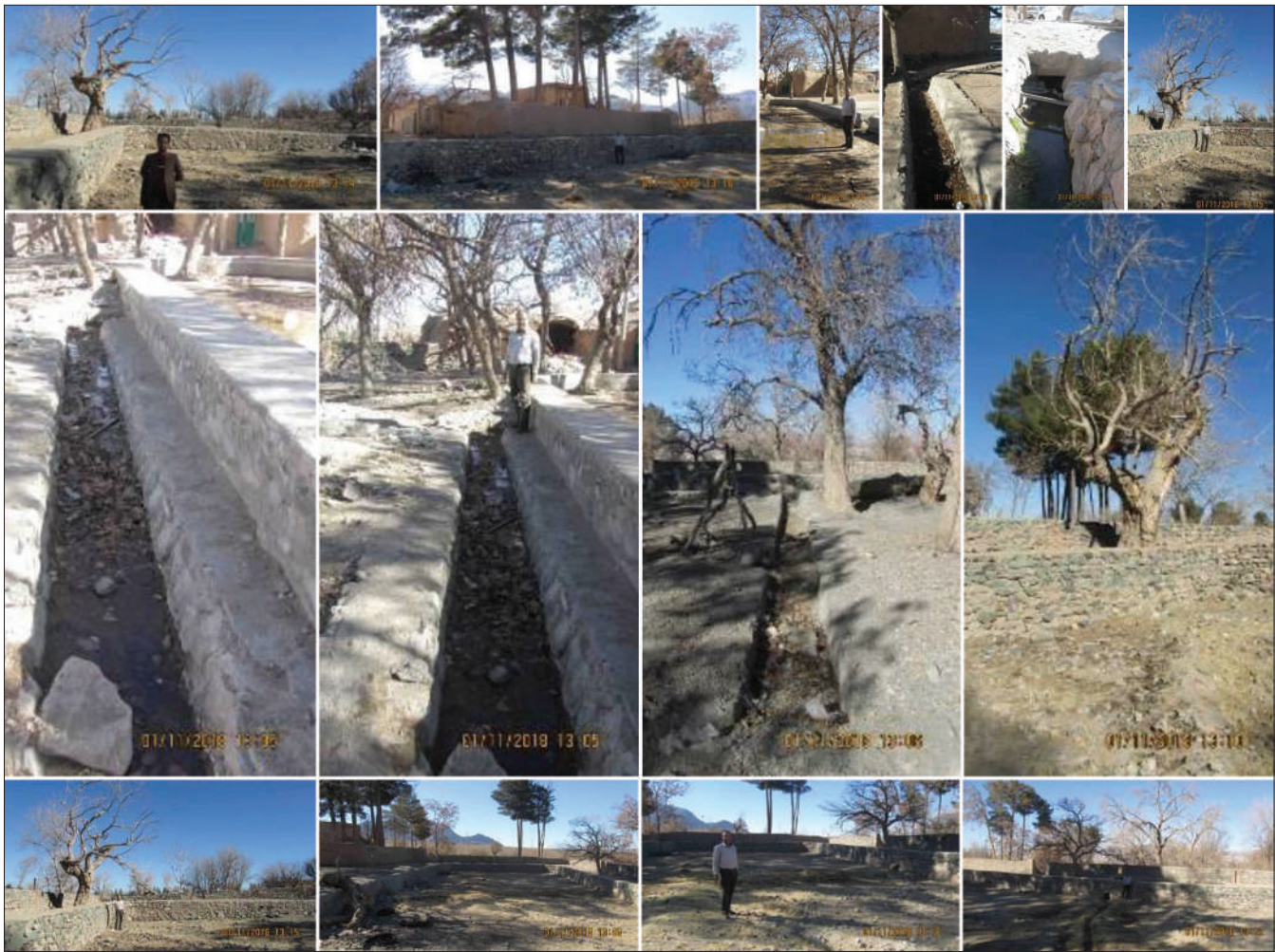
Figure 5: Visiting of author from rural regions in South Khorasan and their aqueducts (qanats) repairing and reconstructing plus dried aqueducts (qanats) that caused migration local people from their villages to cities and urban regions (Establishing a pool for storage aqueduct water in foothills for utilizing by poor villagers and their herds. With author presence in Derakhte Toot village, 180 km. distance to Birjand, center of South Khorasan province, Autumn 2017. Plus, Noforest village, 40 km. distance to Birjand, center of South Khorasan province, and its aqueduct and a pool for storage aqueduct water and villagers with their gardens and cultivating rose for extracting rosewater etc. Spring 2016. Plus, establishing an irrigation canal for transferring aqueduct water to farms of villagers, in about 20 km distance from Birjand, center of South Khorasan Province, 2011 and 2017. Plus, a dried aqueduct and its two empty water storage pools in Bidokht village and its dried trees and empty of population rural region because of continuous and long run droughts in last two decades, five km distance from Birjand, 22 last pictures, January 11, 2018) (Pictures by author, 2011–2021) [8]
